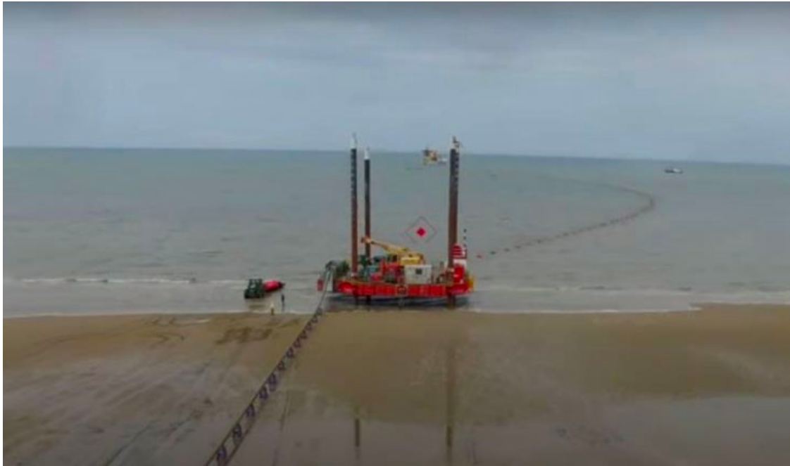
Plate 3.7: Example intermediate pulling platform barge
