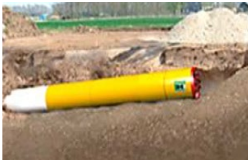
Plate 3.5: MTMB machine at exit location
